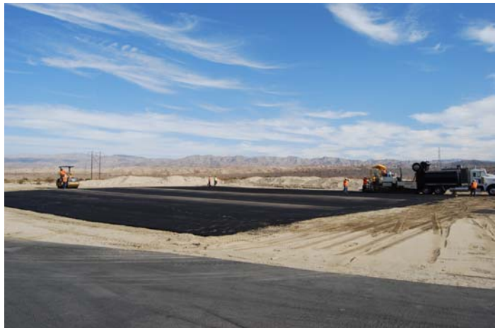
Asphalt U-control apron at North end of parking area.
