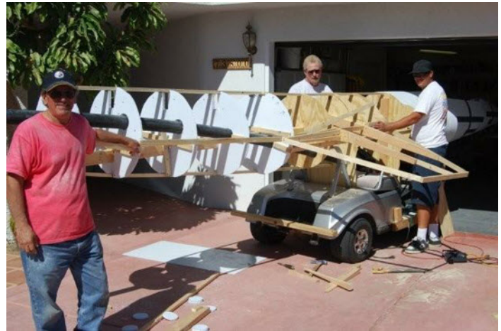
Photo 2, Stringers in place.
